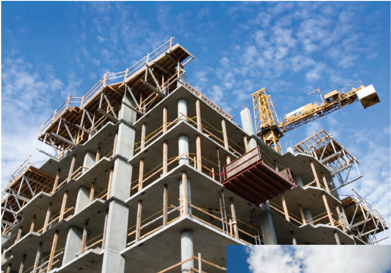
Construction Elevator Emergency Stops
